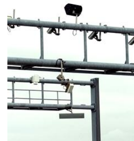
Figure 12: Overhead AVI Antenna [19]
